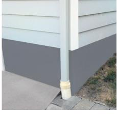
than ground level. You'll be painting below that level so clean it. Remove all dirt and dust from the wall. Use a wire brush and blower. Paint will not adhere to dirt, dust, mud or water.
