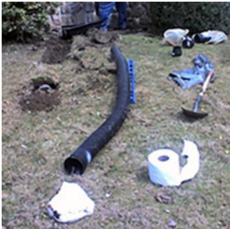
should be off center, indicating down hill, all the way from the house to the end point. The drain pipe will serve a few functions. It will carry (lead) the gutter water away from the house and on its way the pipe will also help to drain the "puddle" areas of your lawn. The pipe needs to be 4" to 6" below the surface of the lawn.
